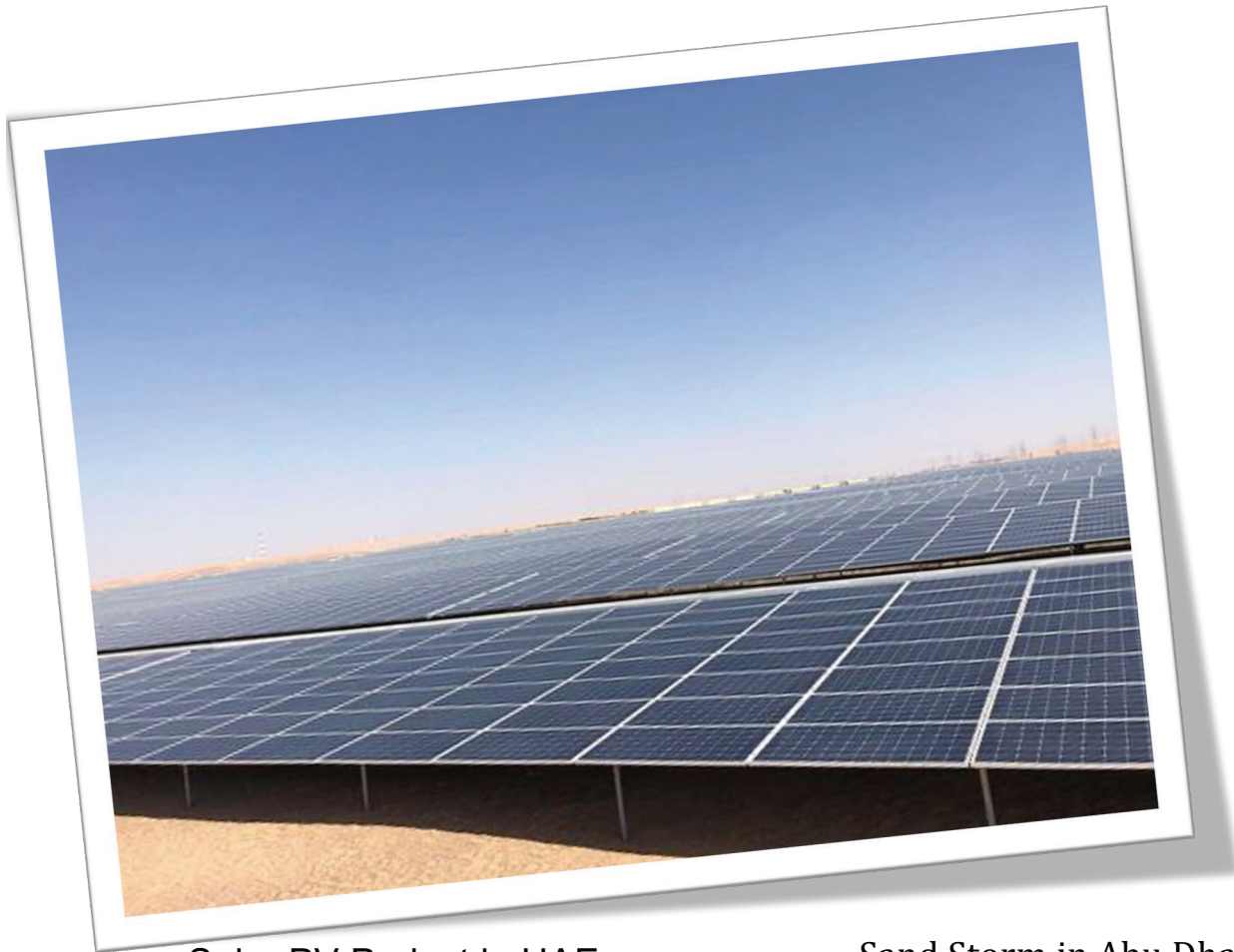
Solar PV Project in UAE
