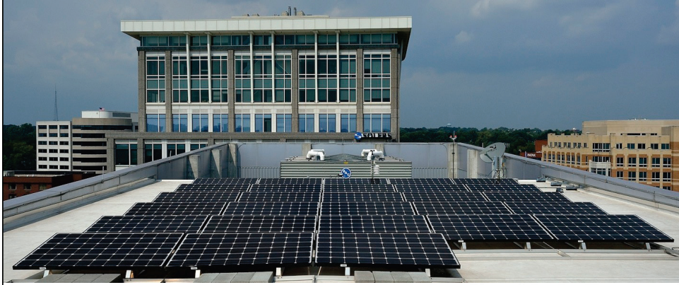
Roof-top Solar at Virginia Tech Arlington Research Center
