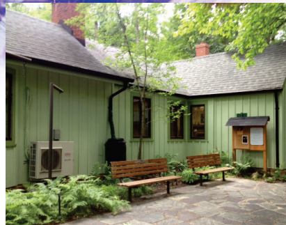
Park facility in Arlington
