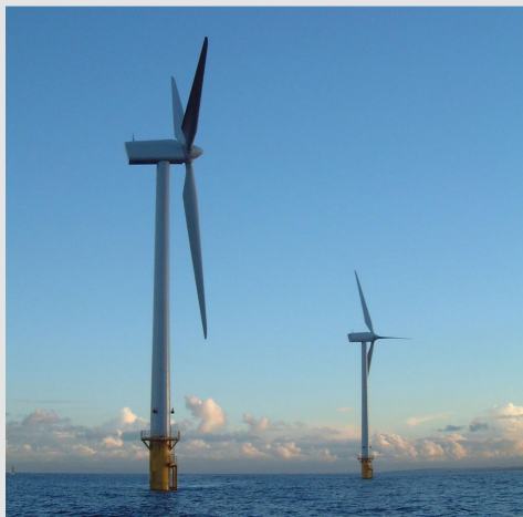
Off-shore Wind turbines, Blyth, U.K.
