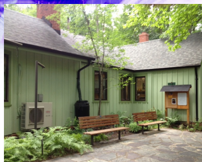
Park facility in Arlington
