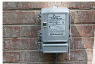
AC Cycling Switch Installed
