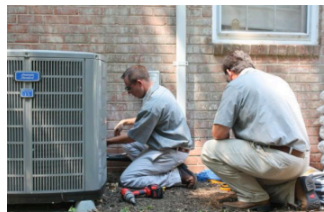
Installing the AC Cycling Switch
